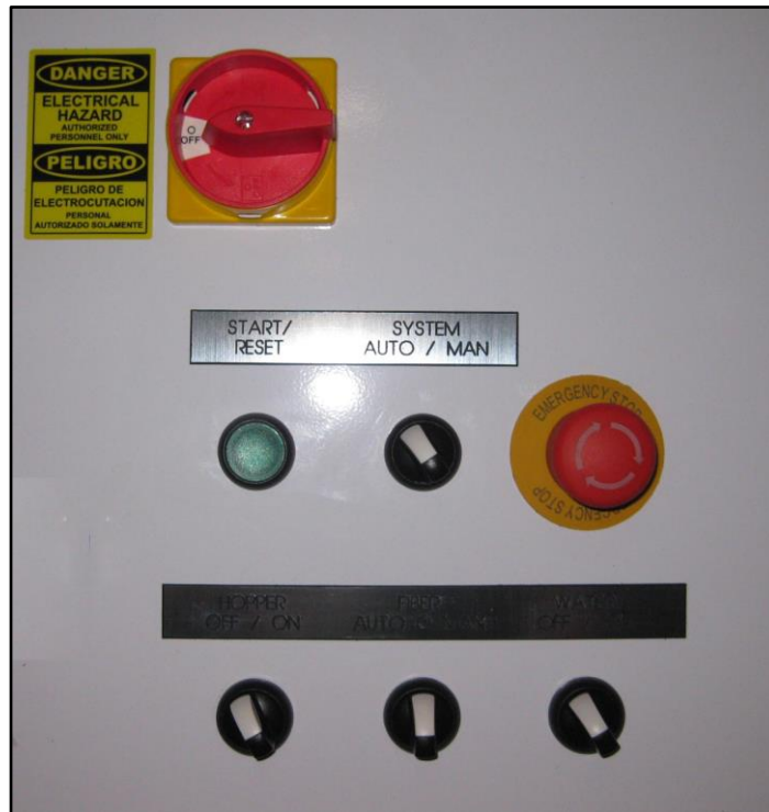
Main controls, electrical control panel door, exterior
